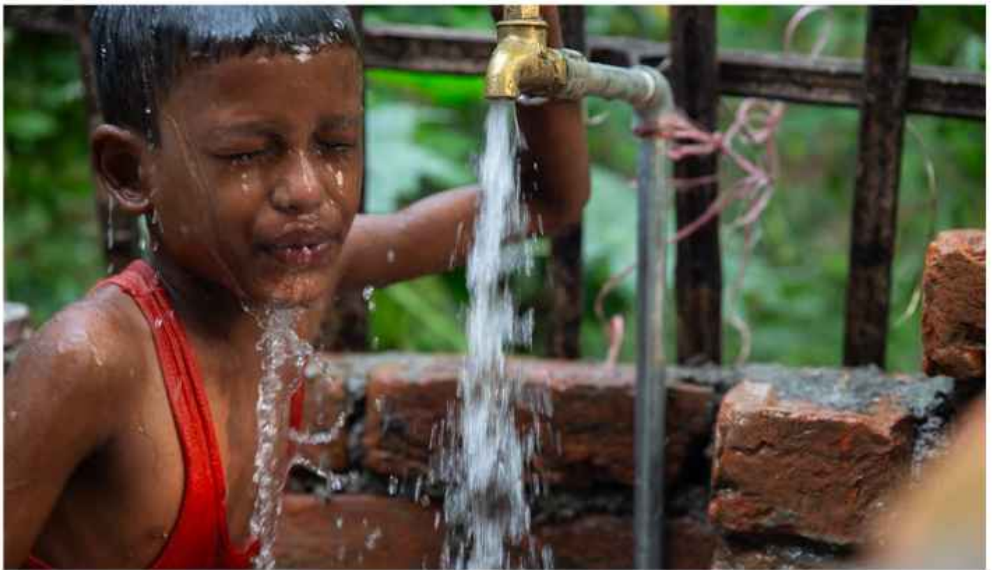
Prashant, 6, starting his day with a quick shower under the newly built tap at his home, Lahan-10, Nepal, October 2023. Credit: WaterAid/Ram Saran Tamang
